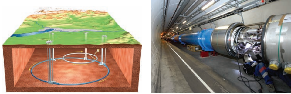
Figure 2.2 The Large Hadron Collider at CERN: a proton–proton collider, based on a 27 km-circle of bending magnets, accelerating cavities and gigantic detectors.
